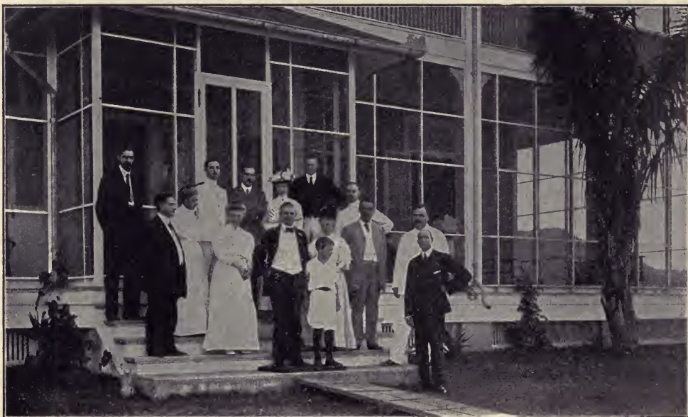
The Residence of Mr. Jno. F. Stevens, Chief Engineer, at Culebra.
