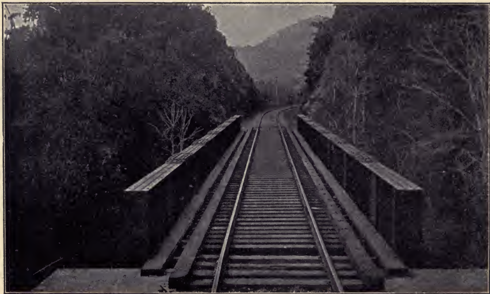
Bridge spanning the Rio Grande.
