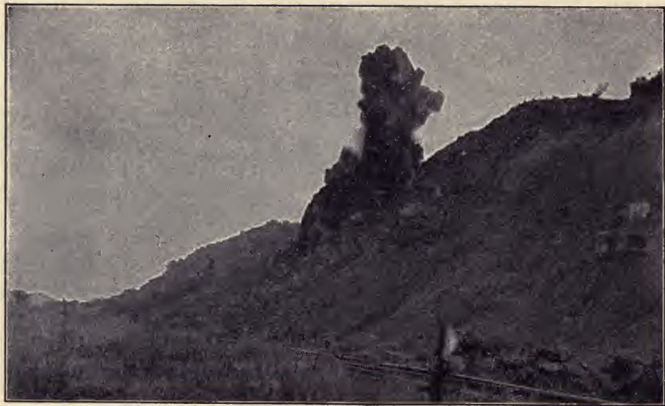
The Great Culebra Cut—a charge of 6,000 lbs. of Dynamite 25 Tons Black Powder going up into the air!
